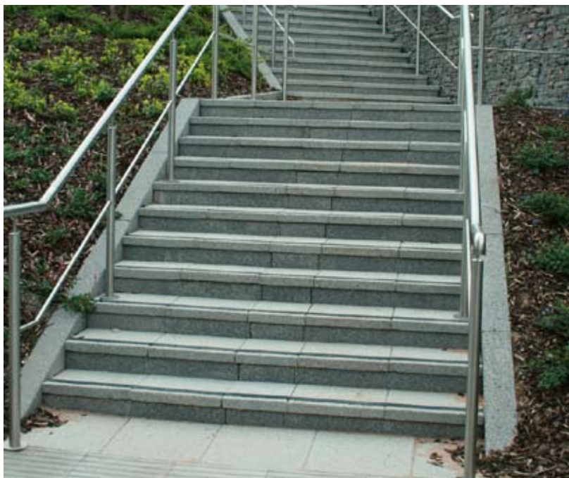
Granite Steps, Hazard Warning Tactile Paving
