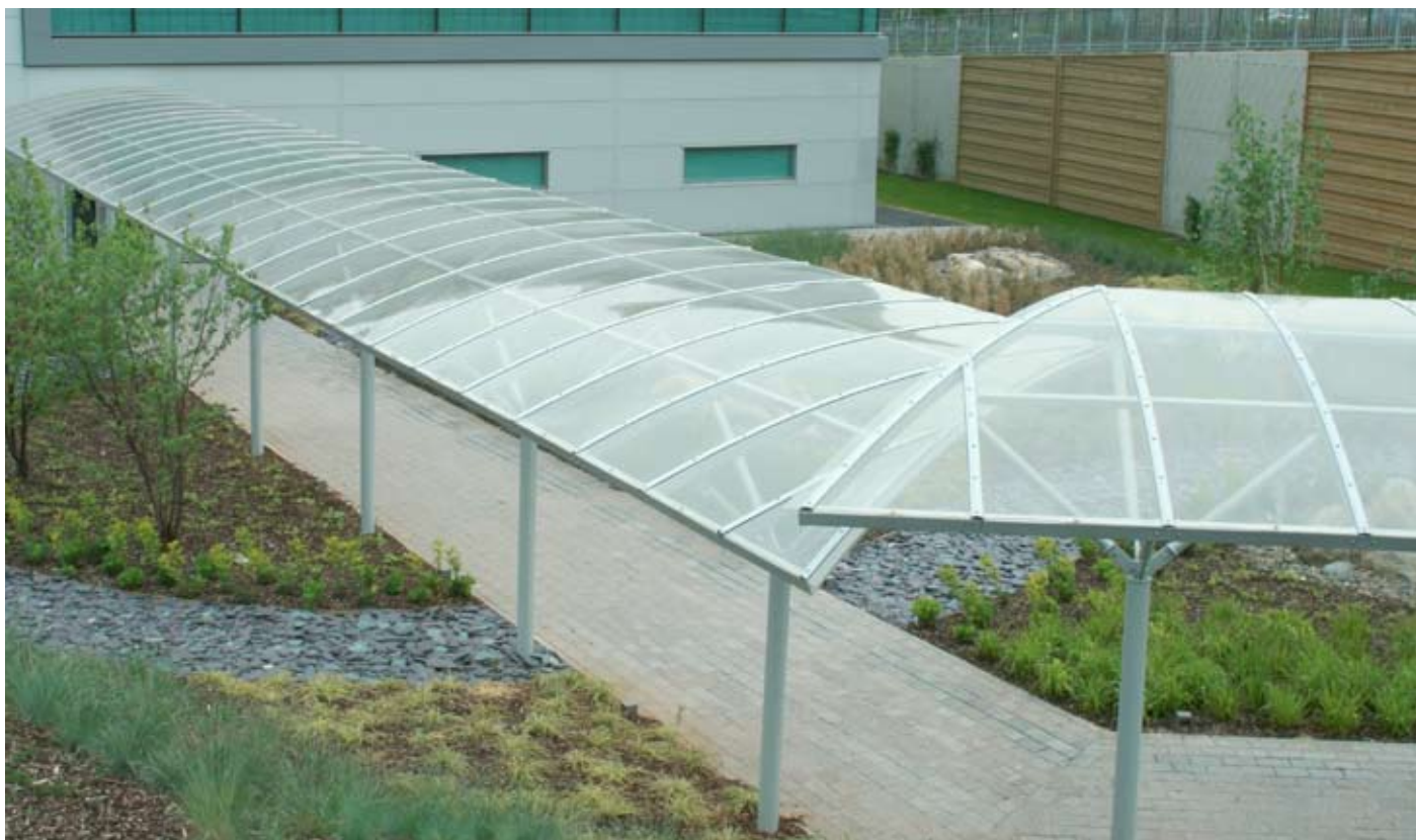
ADI Walkway shields employees from the weather
