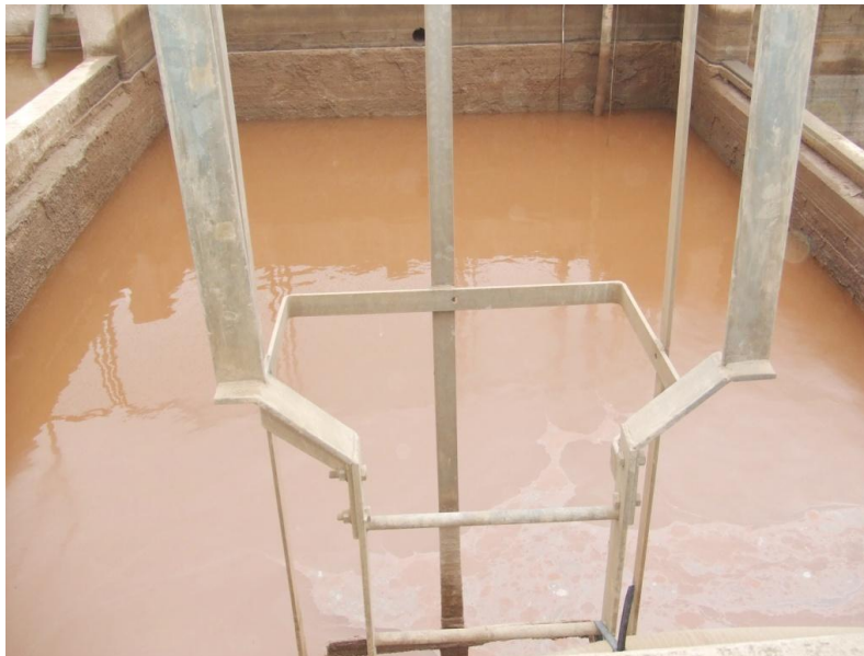
West Lane Works – Stage 1
