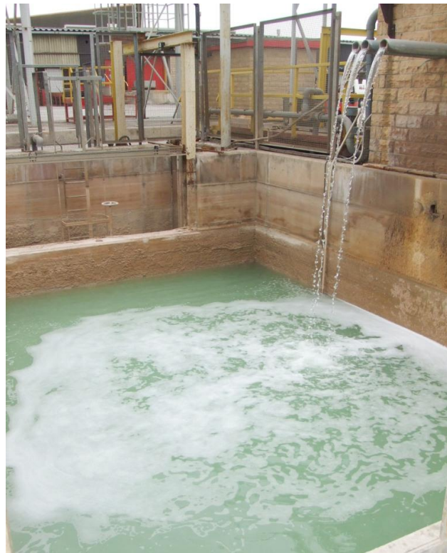
West Lane Works – Stage 3
