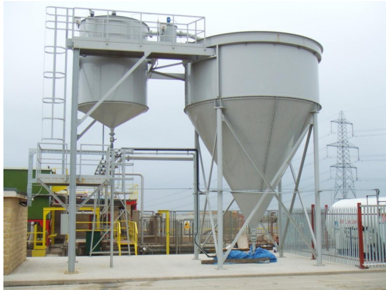
West Lane Works – Stage 2
