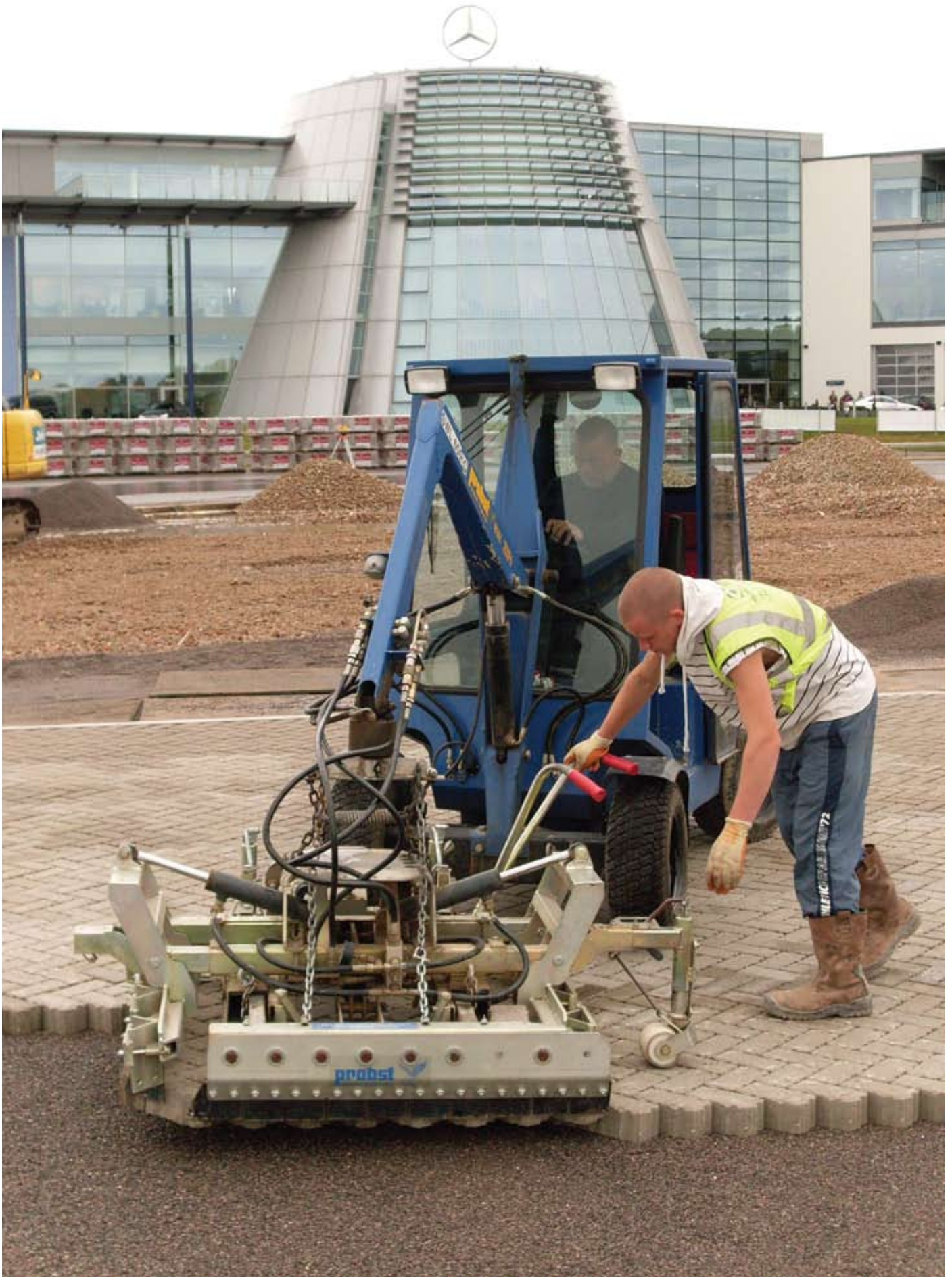
Installation in progress
