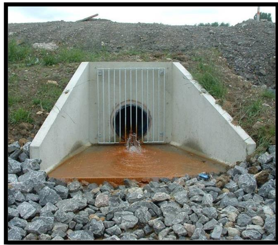
Fig 4 – Marshalls Civils and Drainage Installed Headwall
