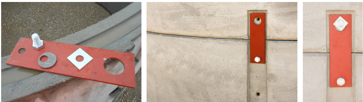
Fig A2 - Joint Connecting Plate
