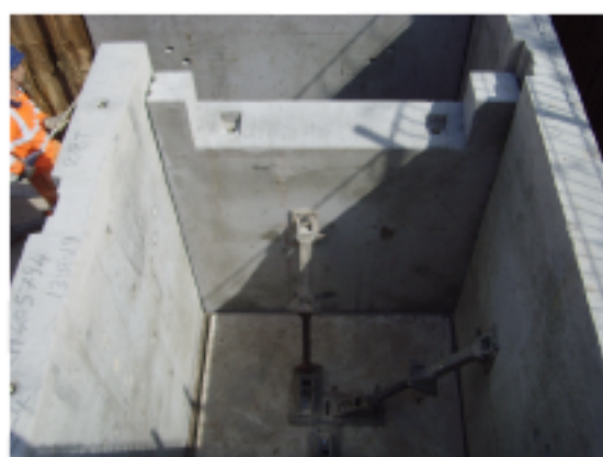
Push pull props to plumb the walls
