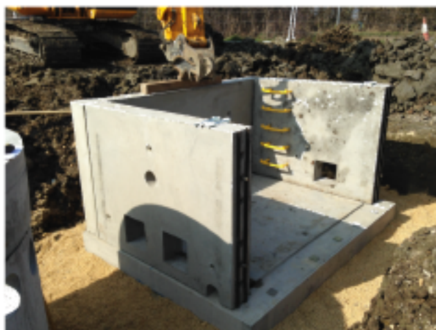
Walls shims prior to placing wall panel
