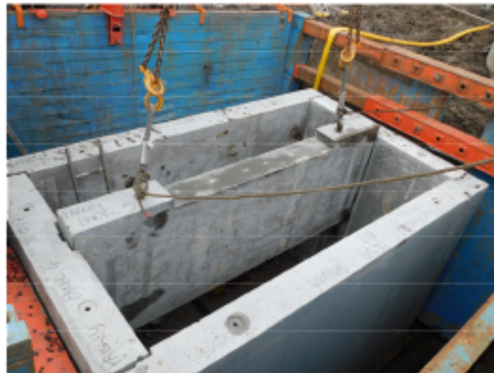
Installing Internal panel
