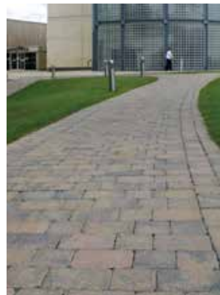
Marshalls Tegula Concrete Block Paving (CBP), Huddersfield University
